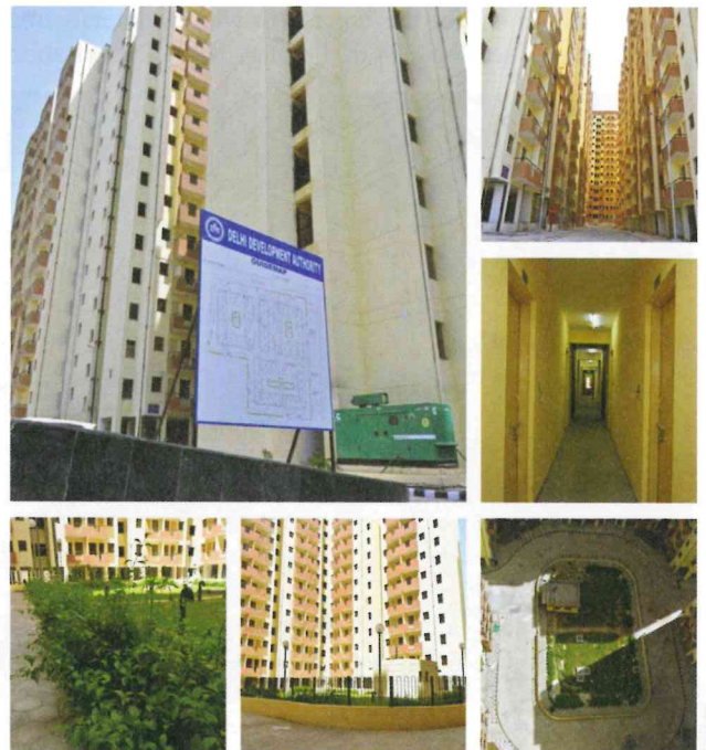
Phase I of the Bhoomiheen Camp, Delhi has 3024 ready-to-move-in flats for slum-dweller beneficiaries
