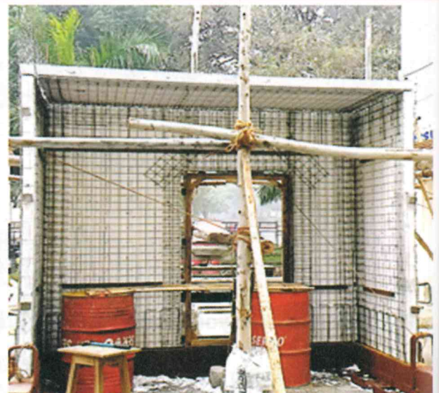
Building skeleton made of factory-made EPS core panels
