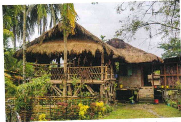
An Adi house has a tall overhanging double roof covering the upper front portion of the house.
