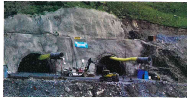
Construction Activity at Zojila Tunnel
