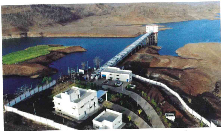
Modern engineering marvel to ensure clean tap water in every home
