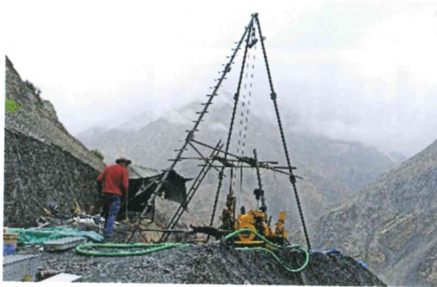
Image 2. Drilling activity by GSI in Himachal Pradesh
