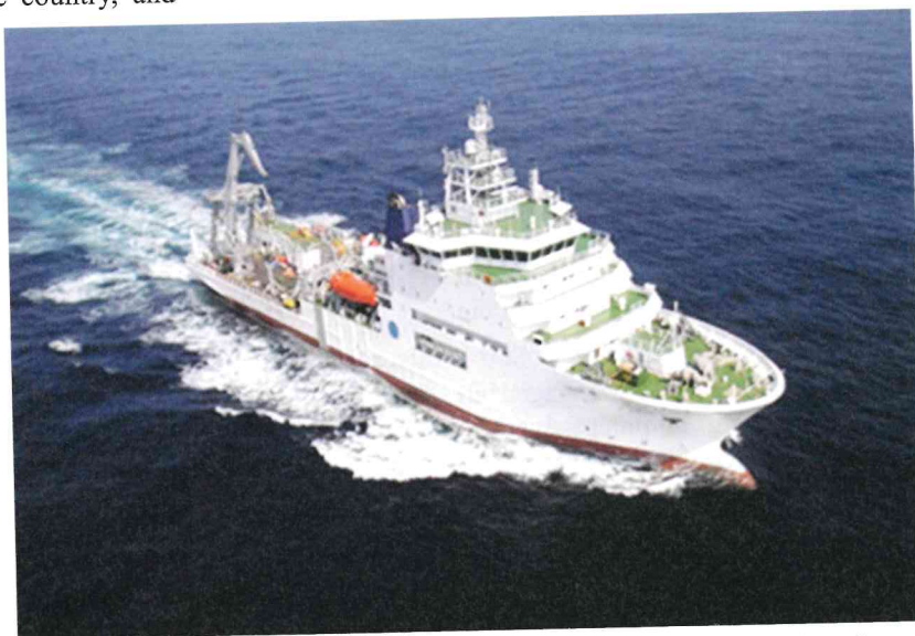
Image 1. Research Vessel Samudra Ratnakar inducted (2013) in GSI's fleet of vessels
